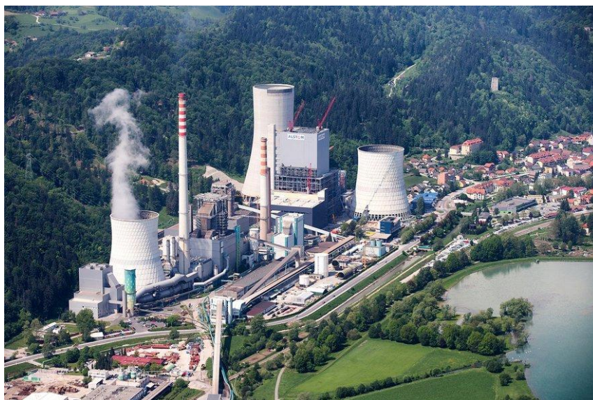
Figure 52: Fossil based power plant in Šoštanj
